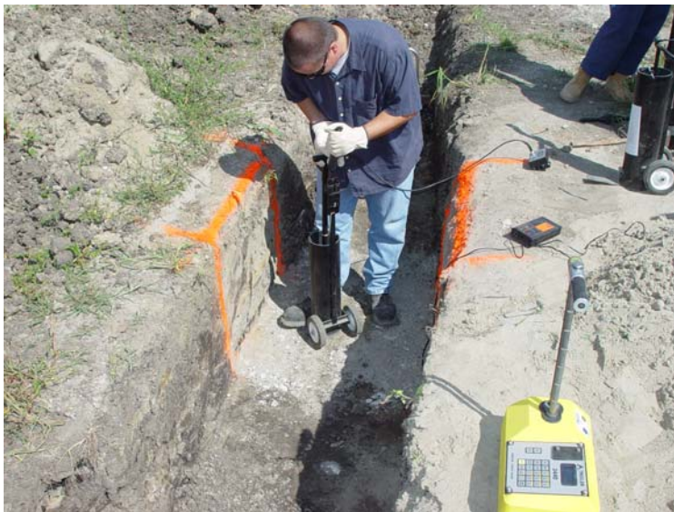
Figure 4 - Use of the Clegg Hammer and NDG in utility trench
